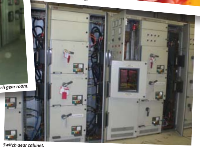
Switch gear cabinet.
