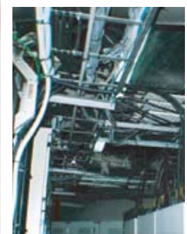
Cable tray at ceiling level
