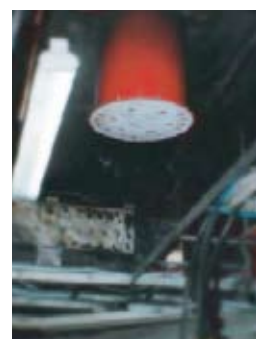
Discharged Pyrogen Generator in front of failed A/C unit
